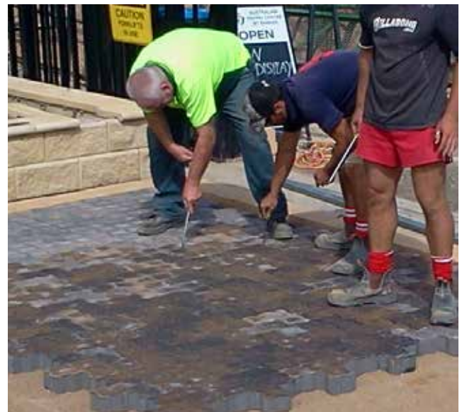
Spacing the pavers to keep straight lines.
